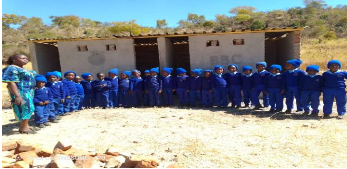
toilets nearly finished
