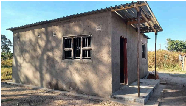
Almost finished. glass,painting etc.
