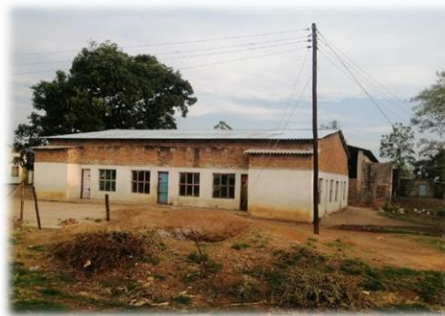
School Roof After Repairs
