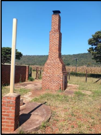
Left: Picture of an Autoway Pit and Chimney that will be built
